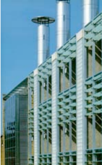
Active facade for natural ventilation
